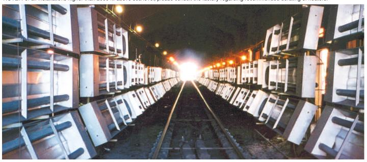
122 RSTP17s installed at a railcar thaw shed of a steel company in IN. The company reported annual savings in excess of \$500,000 in fuel costs, reduced maintenance and elimination of charge backs from damaged railcars and 5 minute cycle times at design temperatures.
